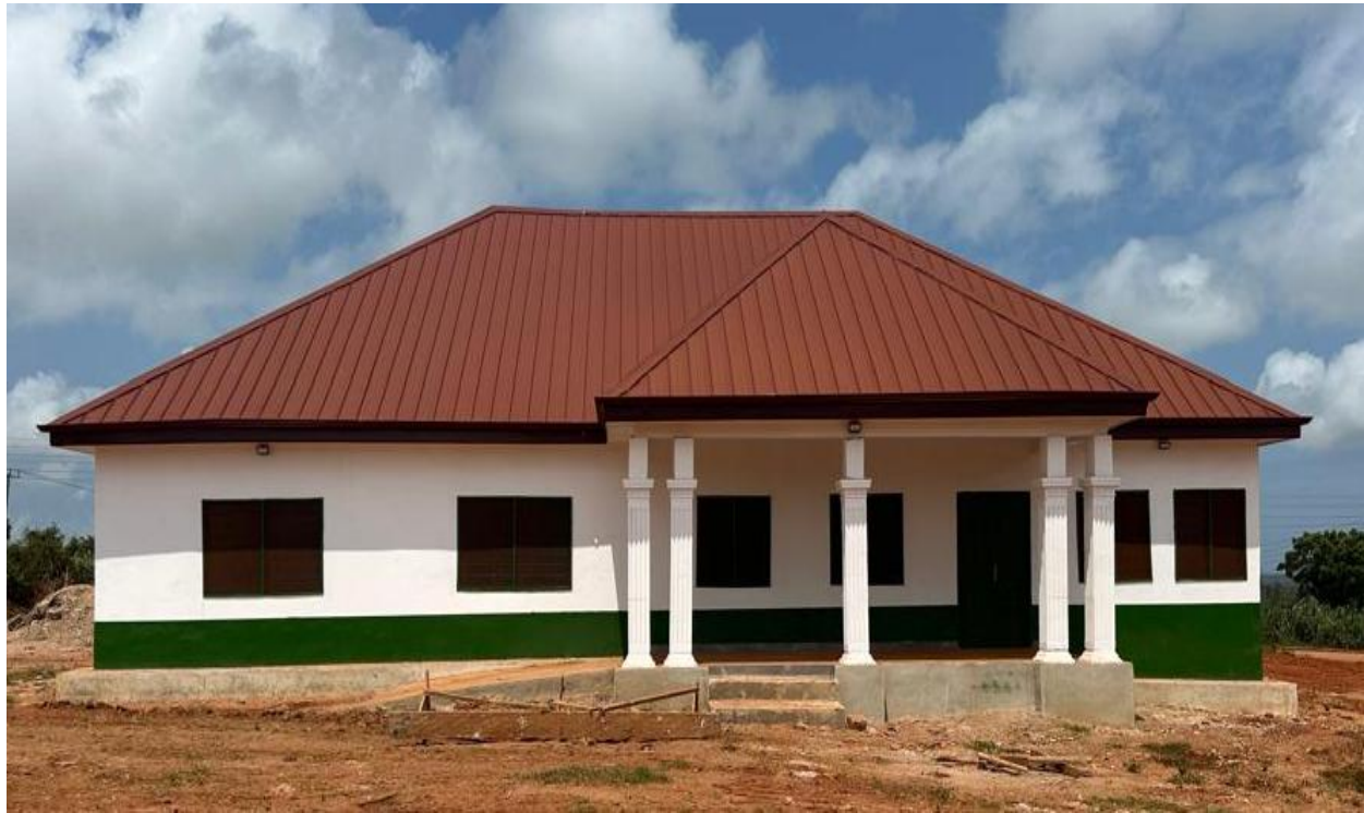
Figure 6: Completed 1no. CHPS Compound with 3-unit Nurses' Accommodation at Ankamu
