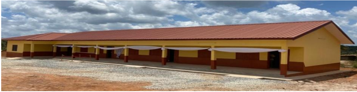
Figure 2: Completed 1no. 2-unit KG Block at Antseadze
