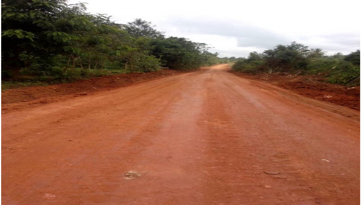
Figure 5: Reshaping of 60.35KM feeder roads within the district
