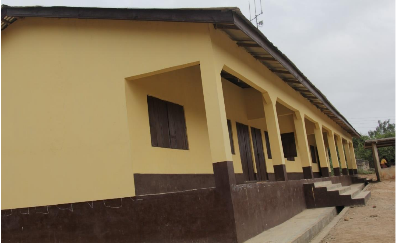
Figure 1: Completion of 1No 3Unit Classroom block with KVIP at Gomoa Obiri
