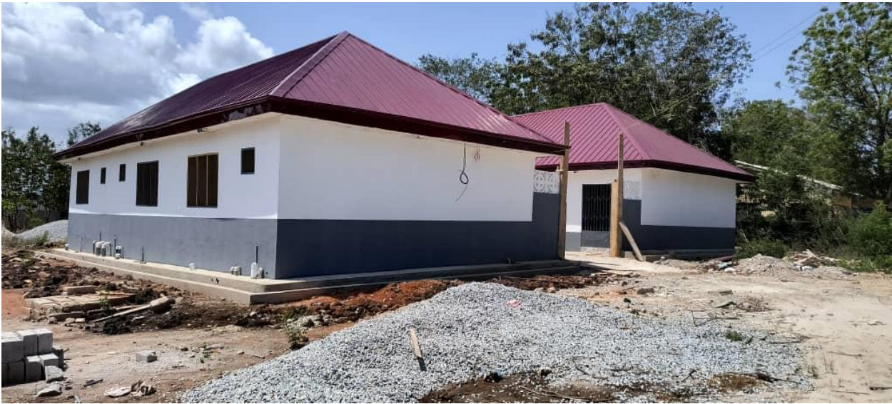
Figure 8: Completion of 1no. 6-unit Teachers' Quarters at Apam.
