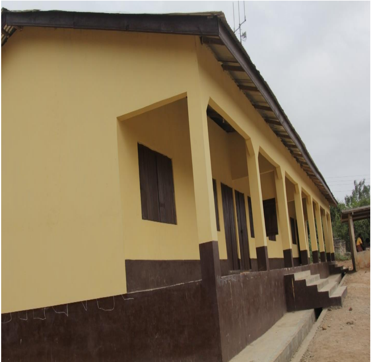
Figure 1: Completion of 1No 3Unit Classroom block at Gomoa Obiri
