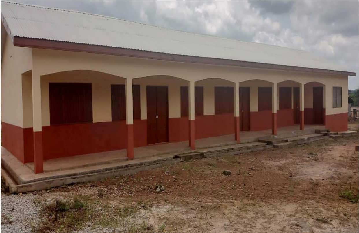
Figure 2: Construction of 1no. 3unit classroom block at Appiakrom Debiso
